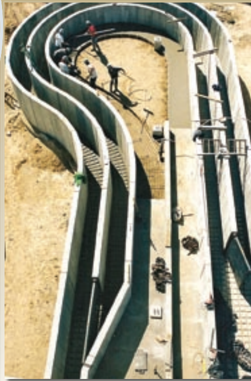
Laying out and pouring the 500-foot serpentine wall for running cattle at a 35,000-square-foot beef processing plant was greatly simplified by using Leica Builder's electronic distance measuring (EDM) device.
