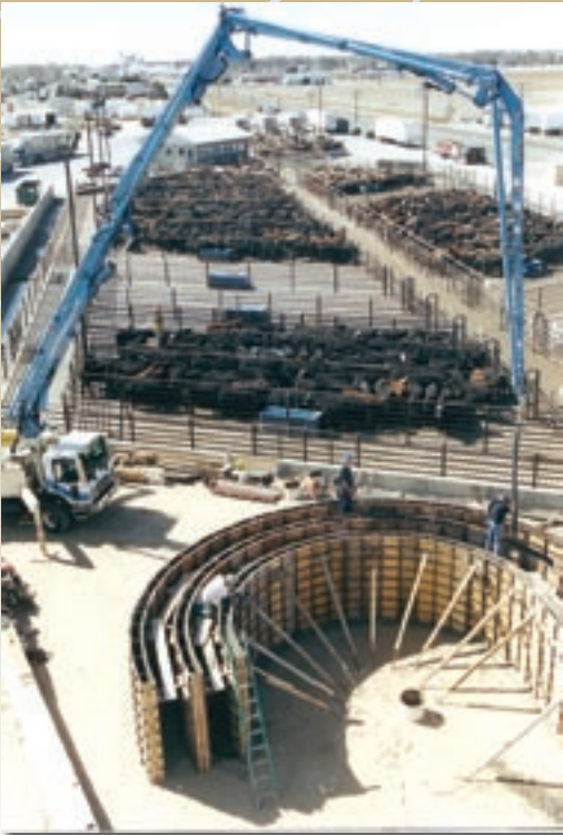
Laying out and pouring the 500-foot serpentine wall for running cattle at a 35,000-square-foot beef processing plant was greatly simplified by using Leica Builder's electronic distance measuring (EDM) device.
